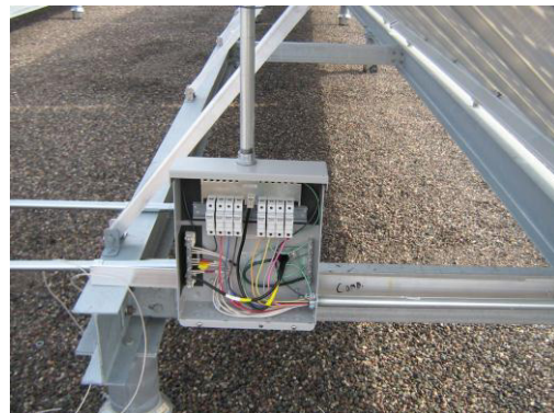
Box lug and screw placement for fuse holder configuration
